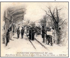
22. Moving platform at the station of the Quai d'Orsay
